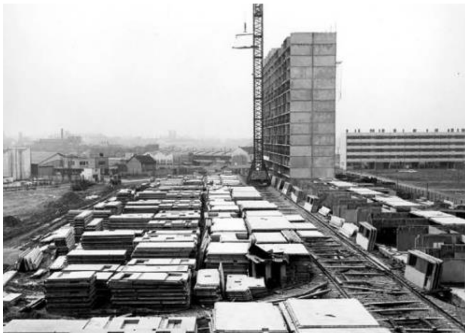
Construction of the 4000s housing estate, Courneuve Paris circa 1957 ( Archives municipales de La Courneuve). The piles of prefabricated concrete panels facilitated the rapid construction of sprawling housing estates.
